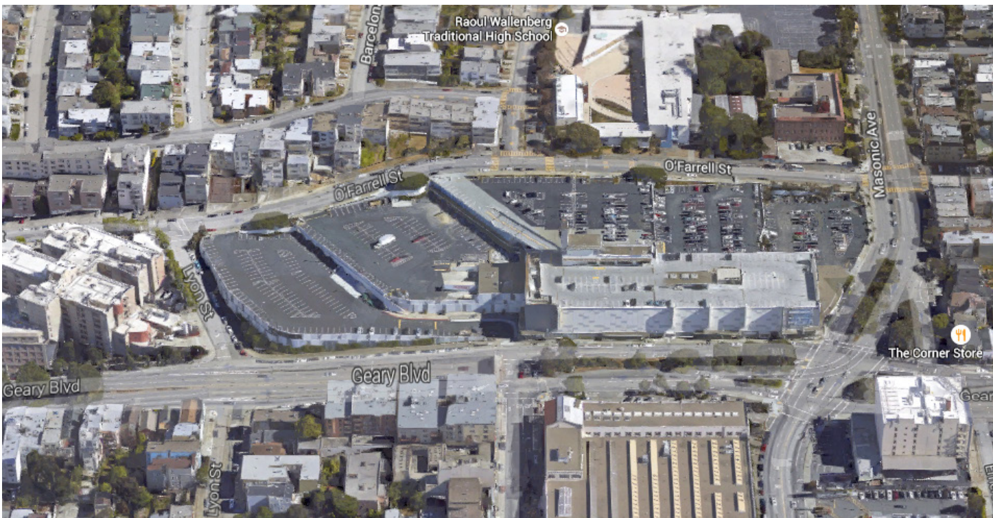
AERIAL LOOKING TOWARD O'FARRELL STREET (FROM NORTH)
