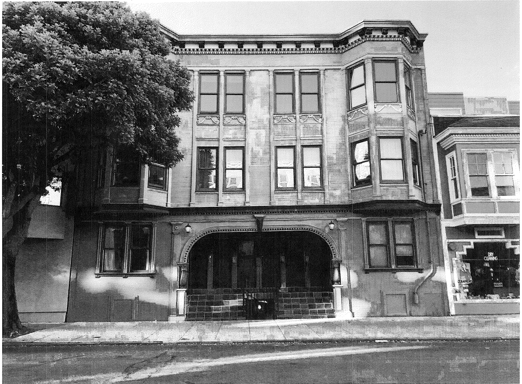
Front of Building
