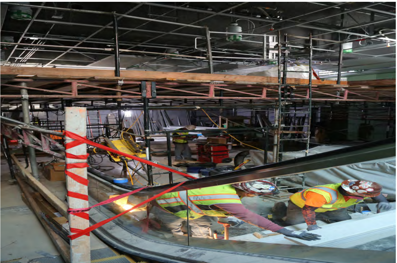
Terrazzo staircase being installed at CTS
