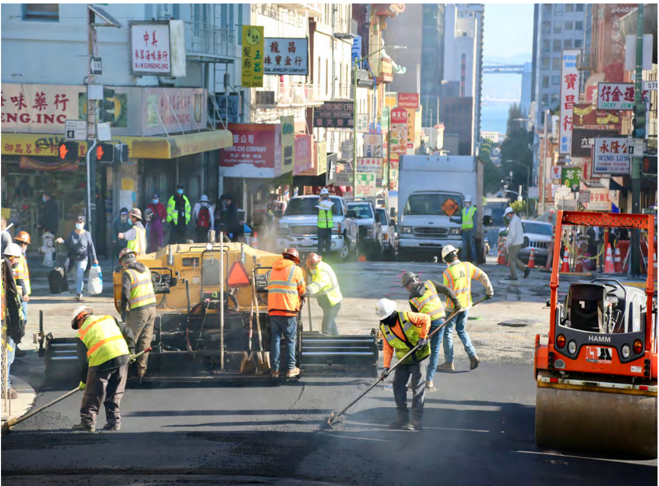
Workers paving asphalt on Washington street.
