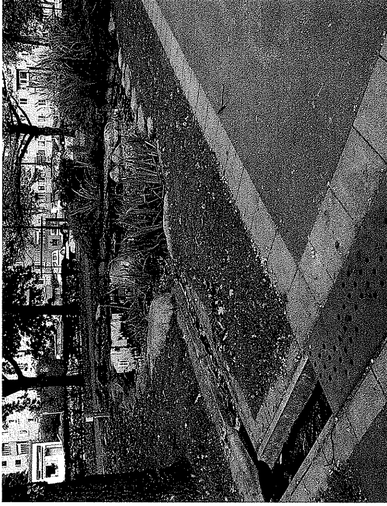
The Ekostaden residential development in Malmö, Sweden, channels all stormwater runoff through BMP treatment features such as bioswales, ponds, and wetlands as shown here. Photo: Brooke Ray Smith
