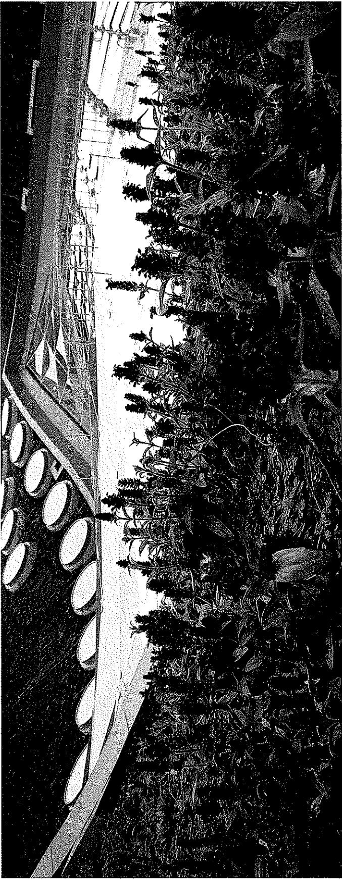
The Academy of Sciences in Golden Gate Park is targeting LEED Platinum certification and includes a 2.5 acre vegetated roof. Photo: Rana Creek - Living Architecture
