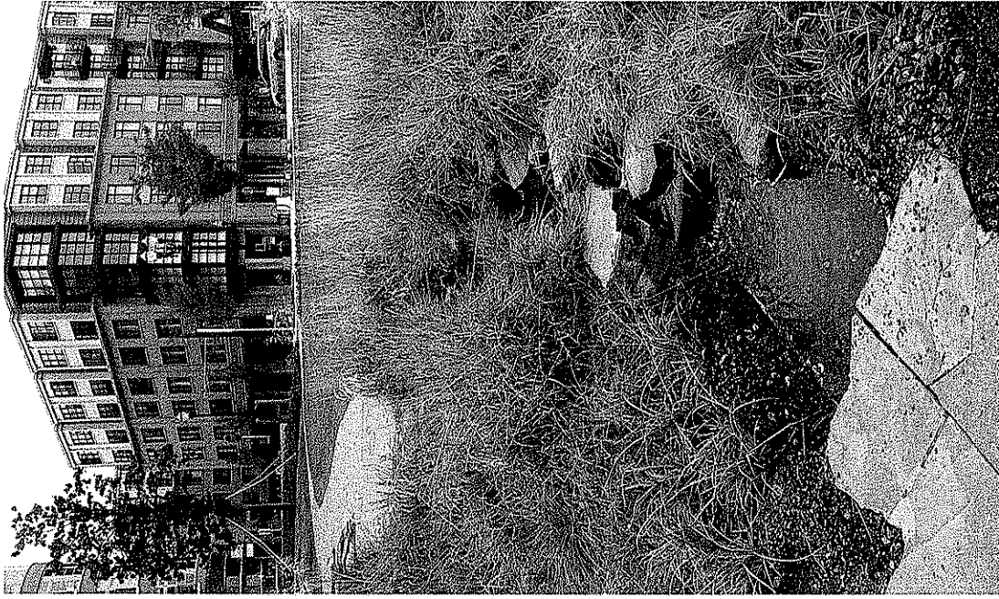
LID measures like the stormwater wetland in Portland's Tanner Springs Park treat polluted street runoff, thereby minimizing negative impacts to water quality.
