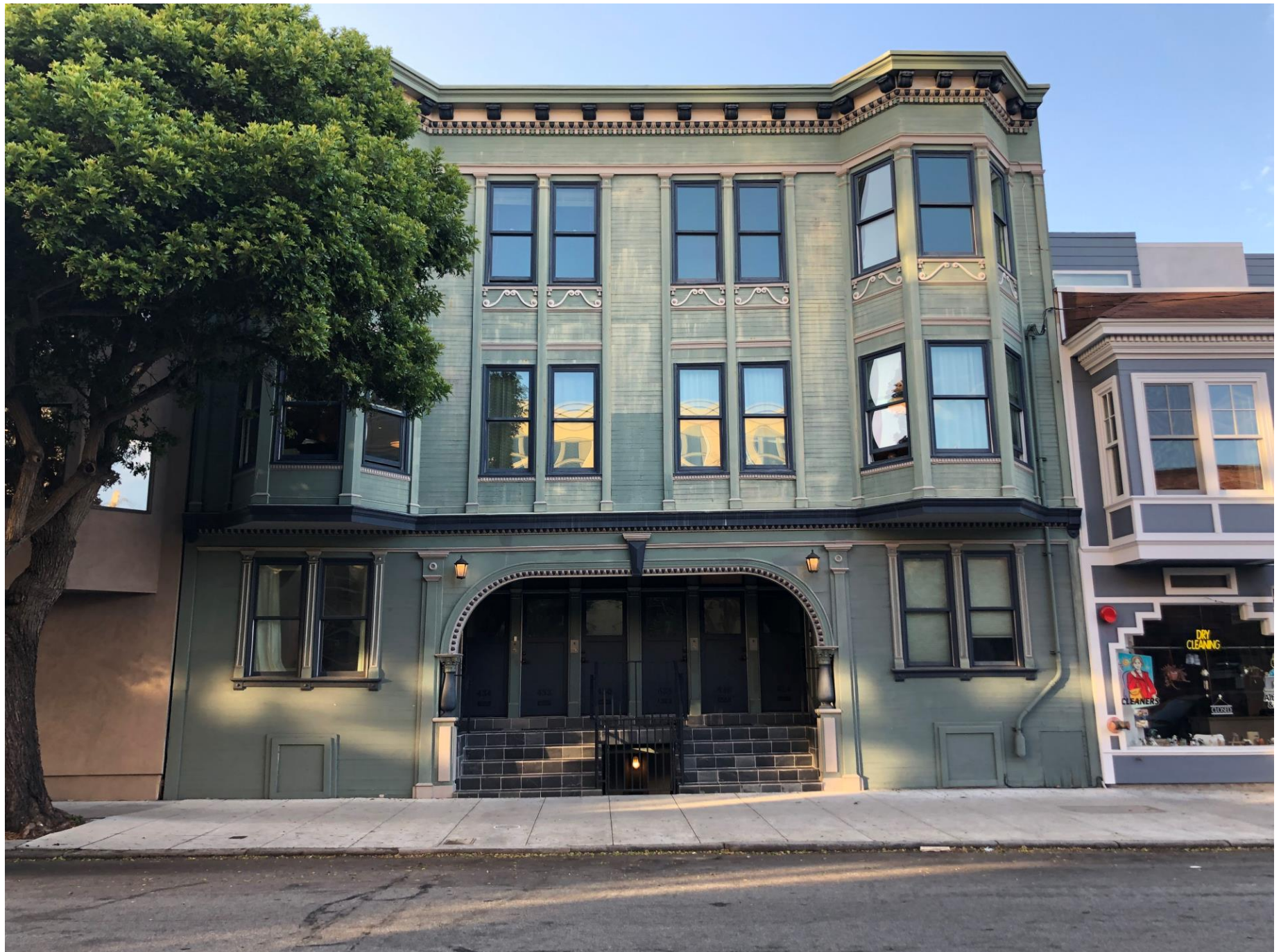
Front of Building
