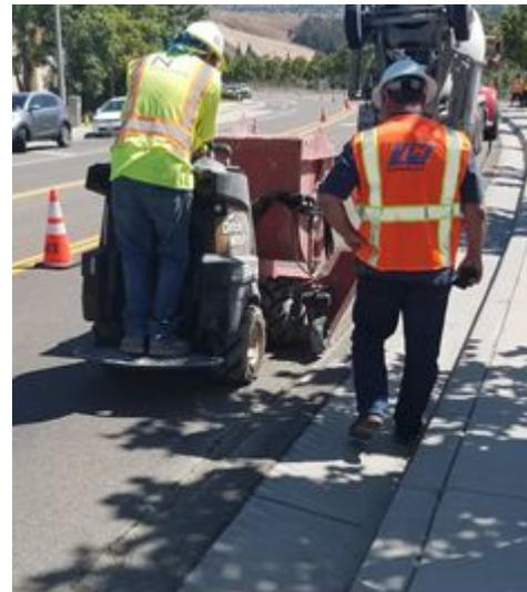
Vacuum unit collects debris. 500-1,000 ft. avg. completion per day.
