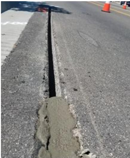
Cement slurry backfill is driveable same day
