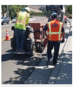
Vacuum unit collects debris. 500-1,000 ft. avg. completion per day.
