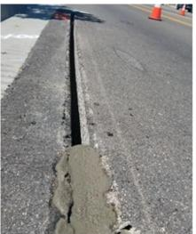
Cement slurry backfill is driveable same day
