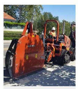
Faster, lower impact method. 16"-24" depth trench cut, 8-9" offset from concrete gutter.
