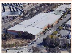
Rehabilitate the Burke Warehouse facility to prepare it for new transit fleet maintenance functions, specifically the housing of overhead lines with increased storage capacity. Work will include the installation of a new roof, new building cladding, insulation, foundation improvements, new lighting, new HVAC systems, and interior improvements.
