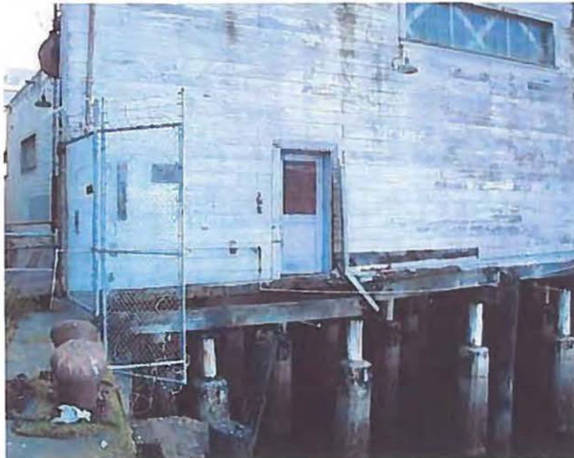
Photo 4: Mandoor exit with no exterior access
