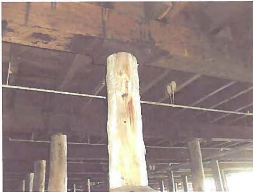
Photo 2: Fungus at Top Pile Section
