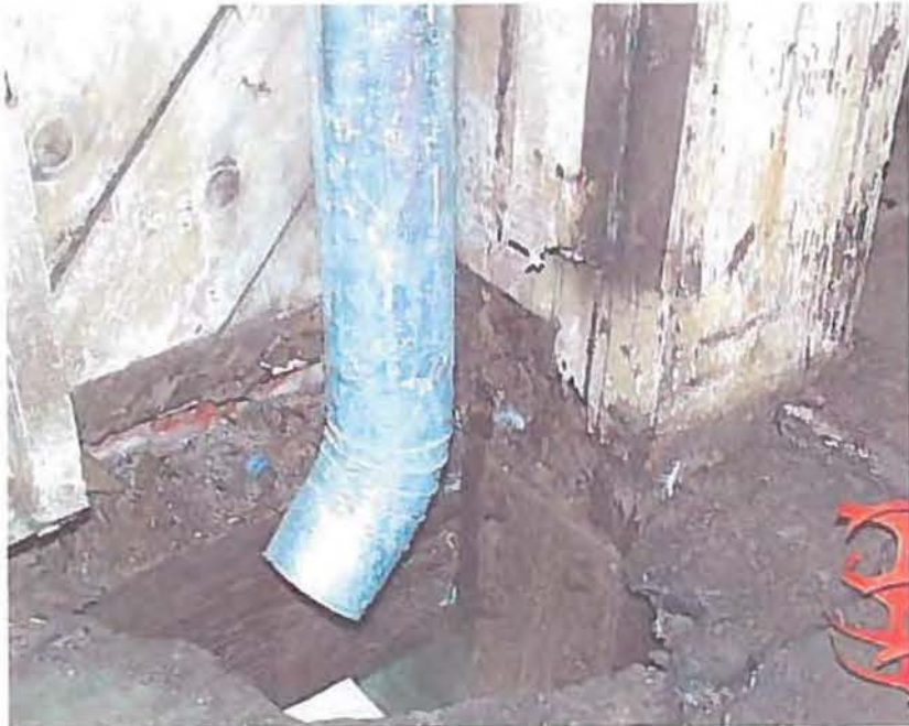
Photo 2: Damaged column base
