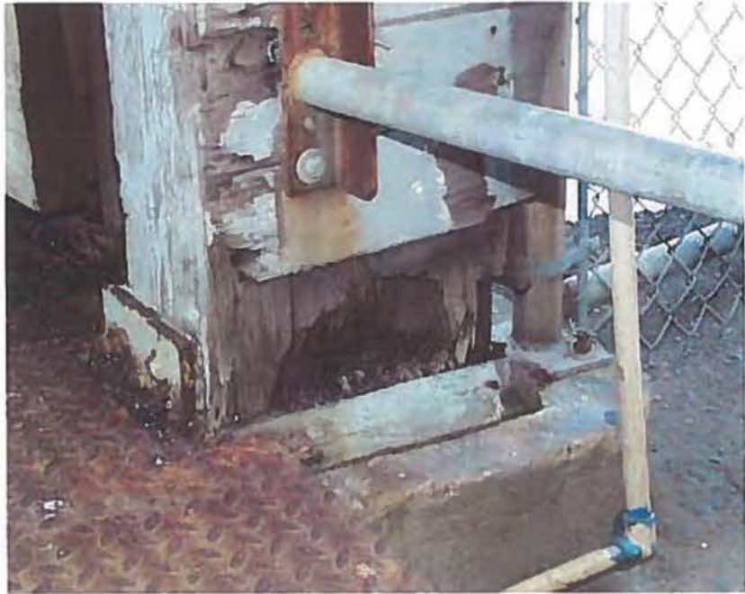
Photo 3: Damaged end wall column base
