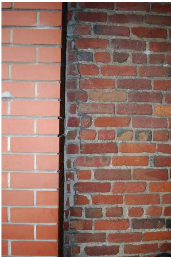
A comparison between the new brick of 1967 (far left) and the old brick of 1906-1907 (at right). This view is in one of the recessed entrances of the main facade.
