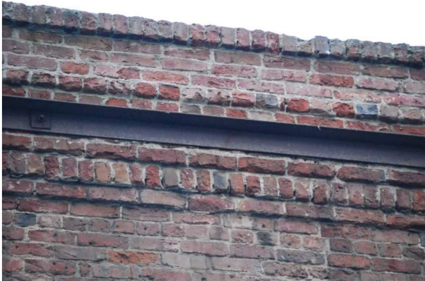
Top left: Rear facade, cornice detail, with added steel reinforcing beam
