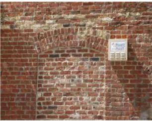
Figure 16. Close-up view of filled-in brick doorway.
