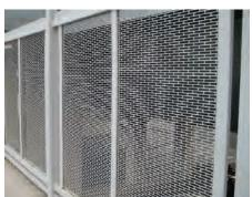
PERFORATED METAL PANEL / GUARDRAIL
