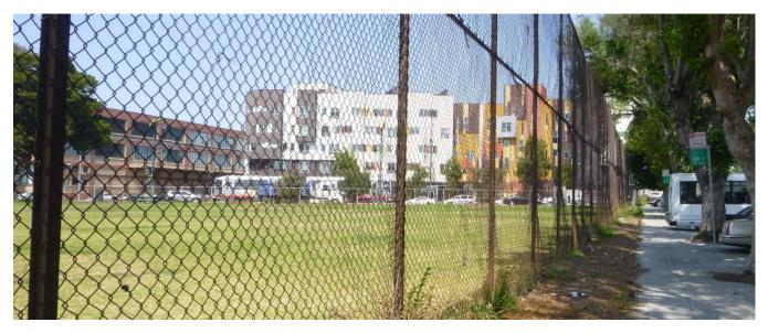
View facing east of the athletic field north fence. The proposed scope is to remove and replace deteriorated fencing fabric, install new gate, and level the surface to create an accessible entrance/exit to the new physical fitness path and athletic field.
