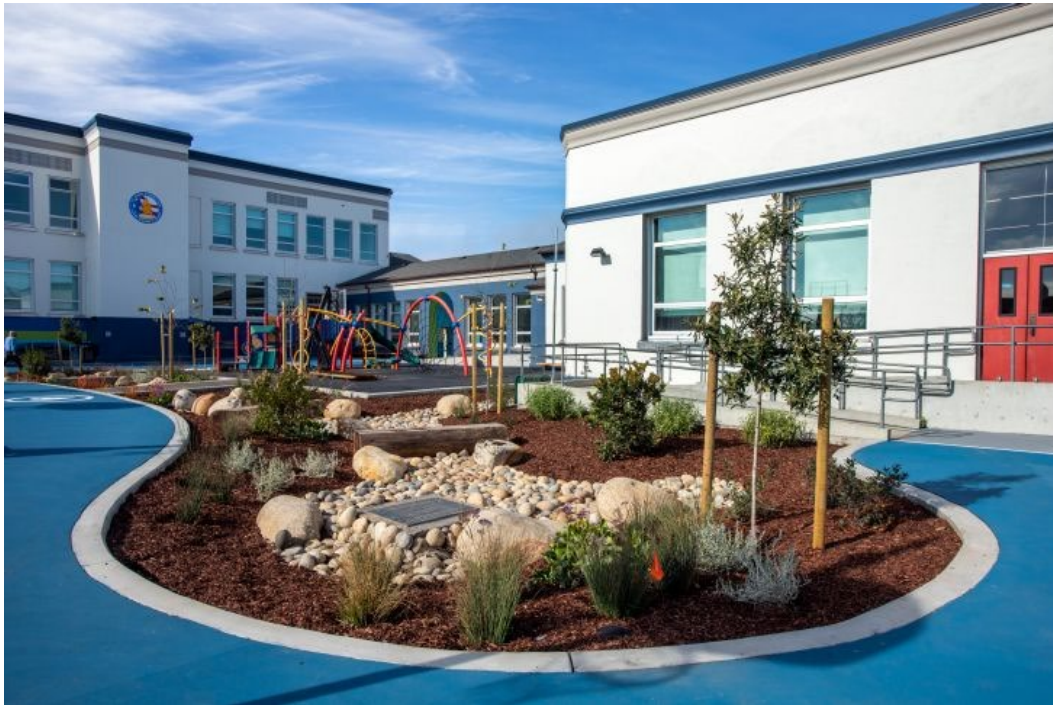
A new Dry Creek Bed in the schoolyard combines nature-play with stormwater management
