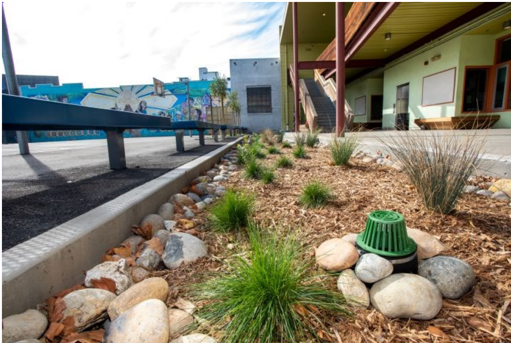
Planters receive stormwater runoff from school roof and blacktop
