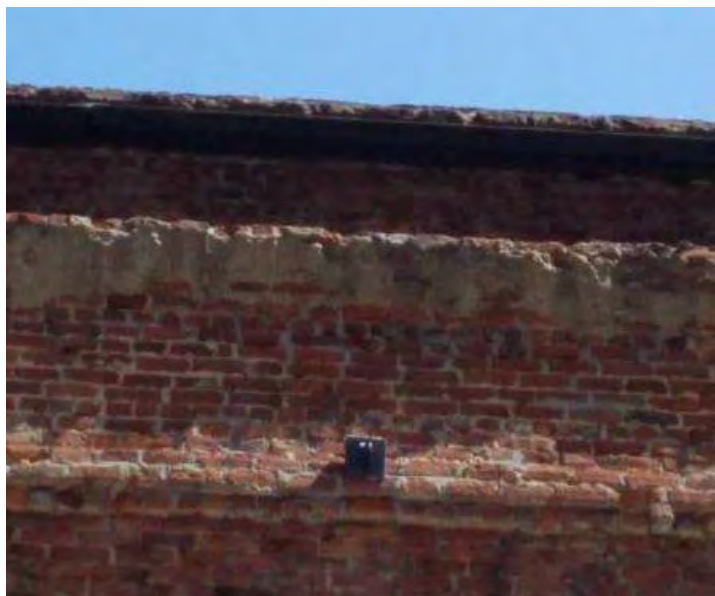
Close up of patched bricks at cornice, 2017. Source: Page & Turnbull, Inc. (2017) report
