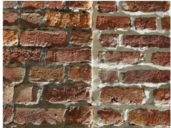
Figure 37. Close-up of bricks showing areas that were recently sandblasted (right) and not (left).
