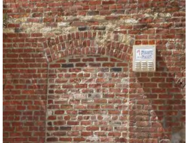
Figure 16. Close-up view of filled-in brick doorway.
